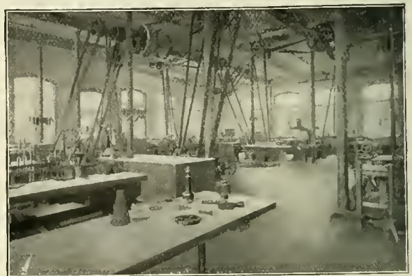
VIEW OF THE PATTERN SHOP.
